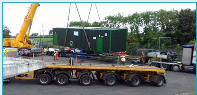
Installation of the modular pumping station.
