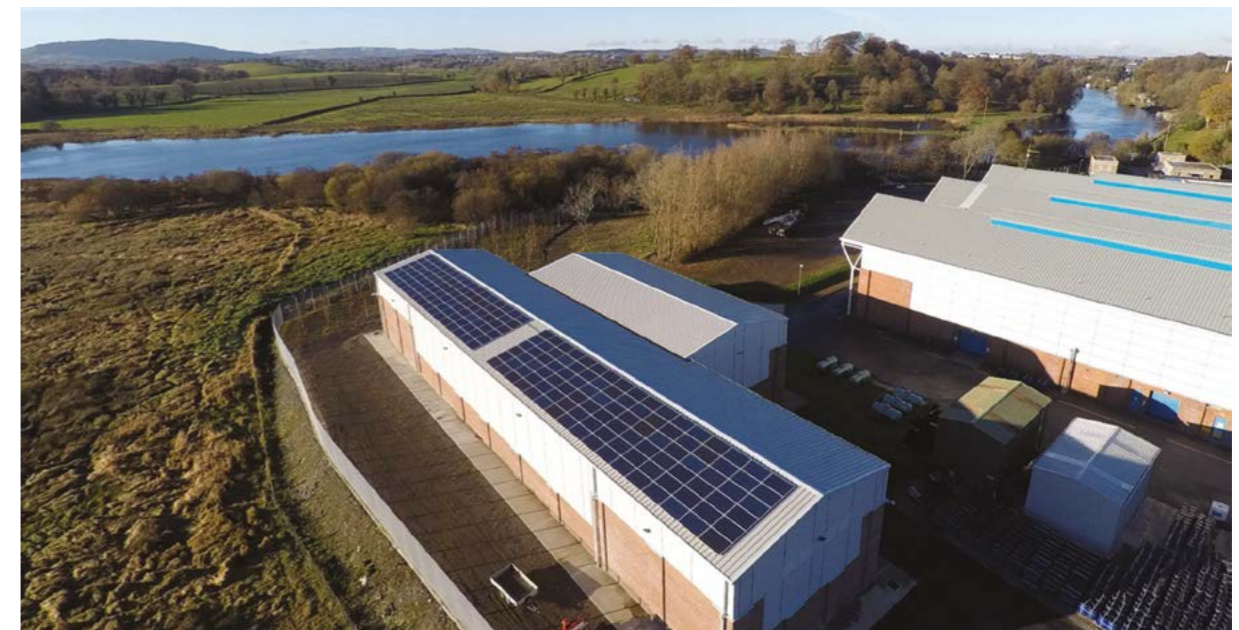
Killyhevlin water treatment works Enniskillen, County Fermanagh.
