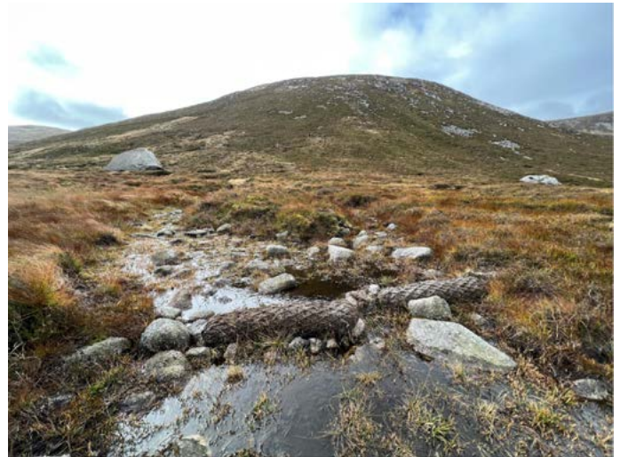
Photo courtesy of Simon Gray, Ulster Wildlife - showing peatland rewetting with coir rolls on Slieve Binnian, Mourne Mountains.
