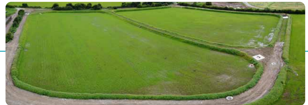
Ballykelly integrated constructed wetland, County Derry/Londonderry
