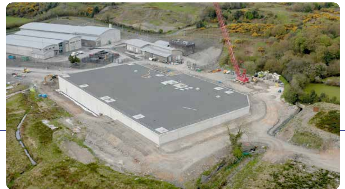
New water storage tank under construction at Drumaroad water treatment works, Castlewellan, County Down
