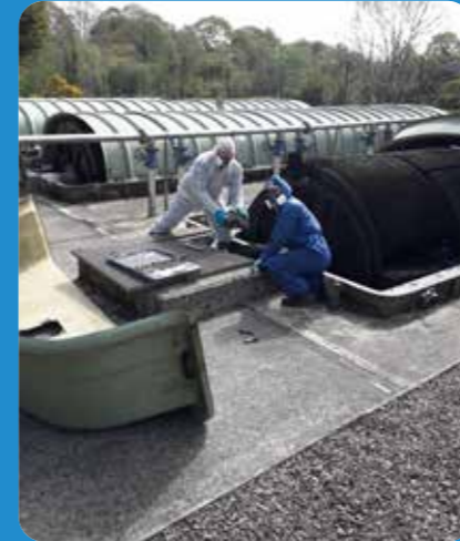
Mechanical and electrical operatives carrying out repairs
