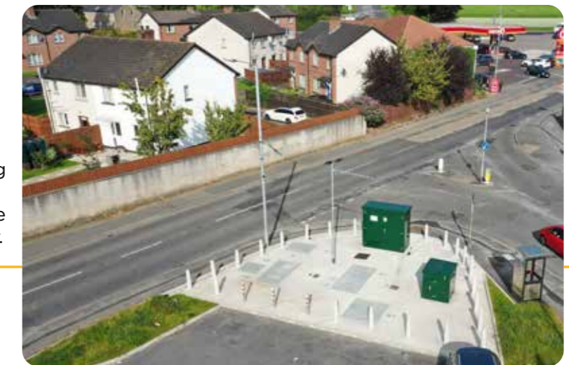
New wastewater pumping station in the west of Armagh City, County Armagh
