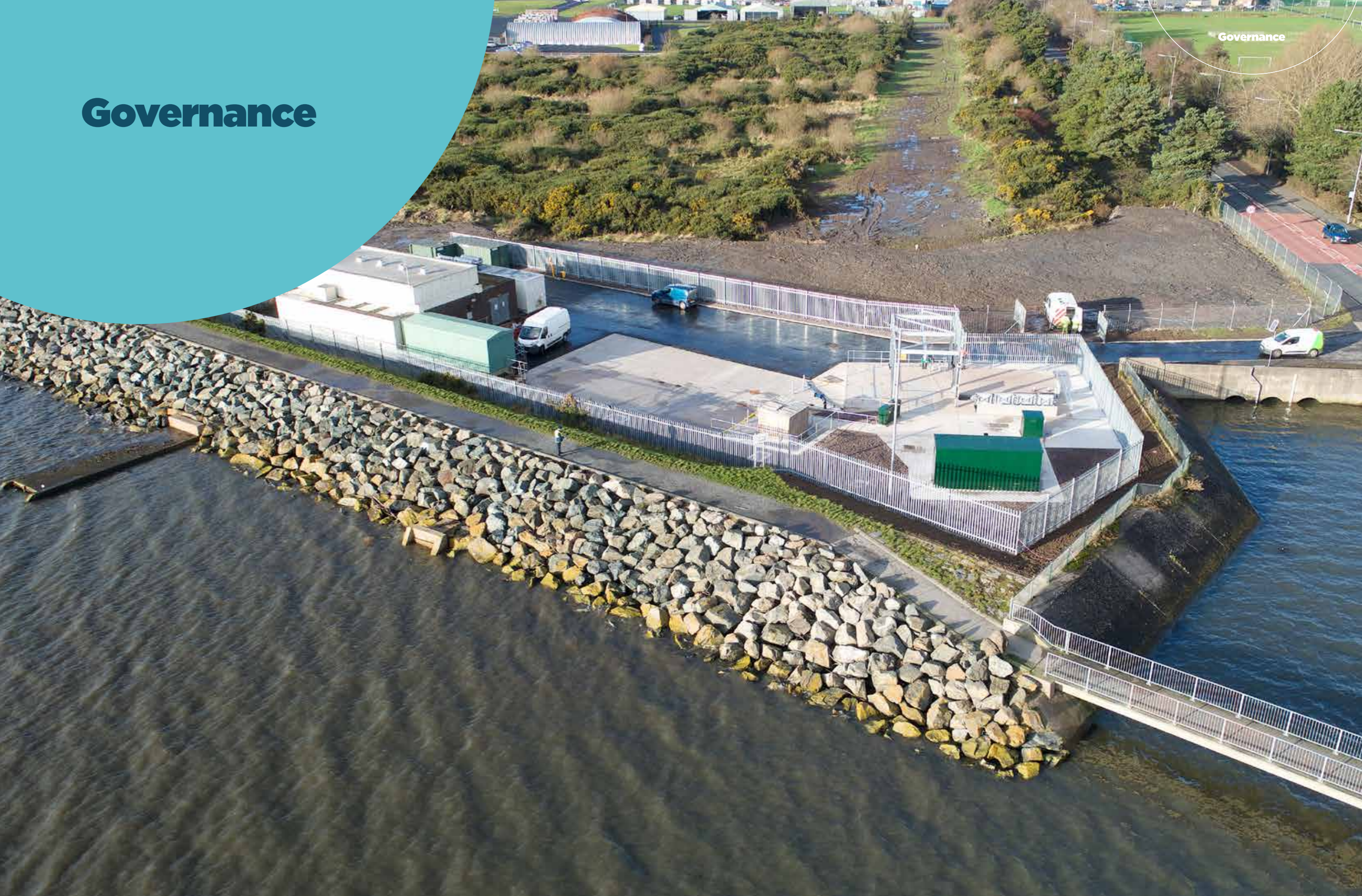
Portaferry Road wastewater pumping station, County Down
