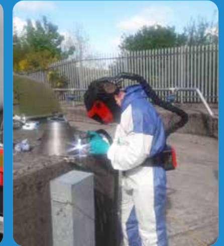
Mechanical and electrical operative repairing a screen
