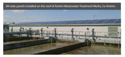
Solar Panels have been installed at Antrim, Lisnaskea and Newry wastewater treatment works as part of a trial. The aim of this trial is to help NI Water understand the potential benefits of this form of renewable energy and evaluate its performance. The panels will provide a reduction of 70,000kwhrs from the electricity grid equating to savings of around £18k per year.
