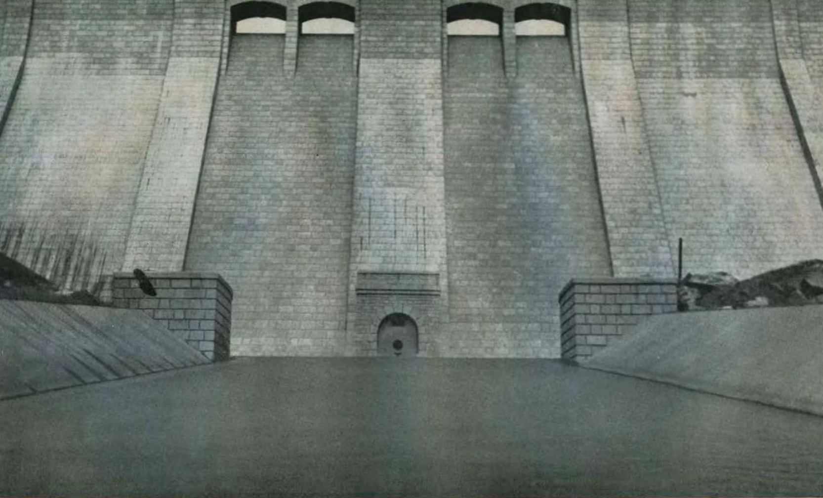
Ben Crom Reservoir Dam
