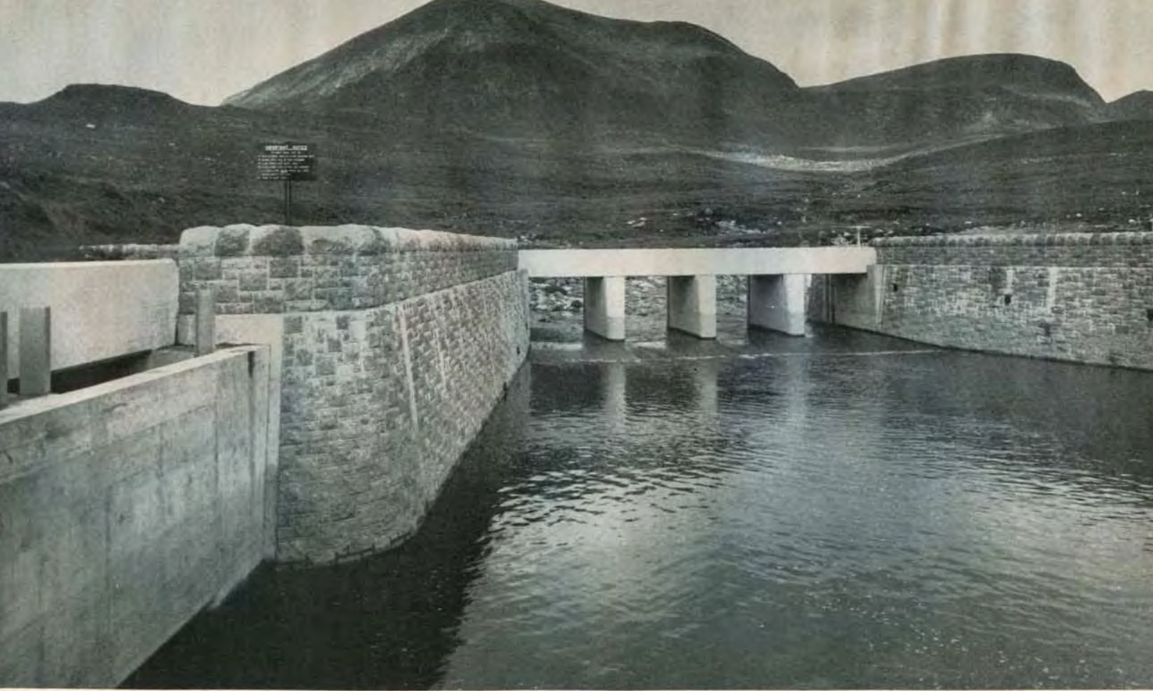
Tunnel Intake Annalong Valley
