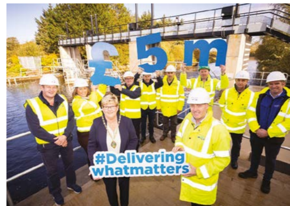
Deputy Mayor of Derry City and Strabane District Council and NI Water and Contractor staff at River Faughan raw water pumping station, County Derry/Londonderry.
