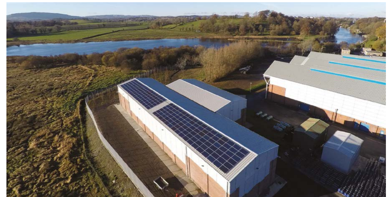
Killyhevlin water treatment works Enniskillen, County Fermanagh.
