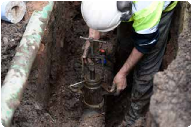
Lead communication pipes being replaced
