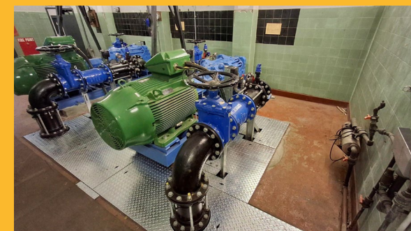
Pump replacement work at Whiteabbey water pumping station, County Antrim.
