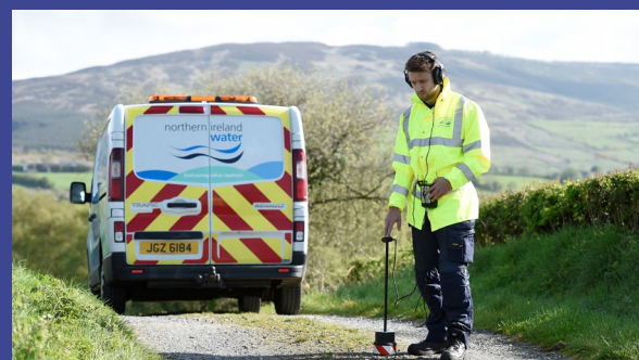
Detecting leaks utilising satellite imagery, handheld devices and ground microphones.
