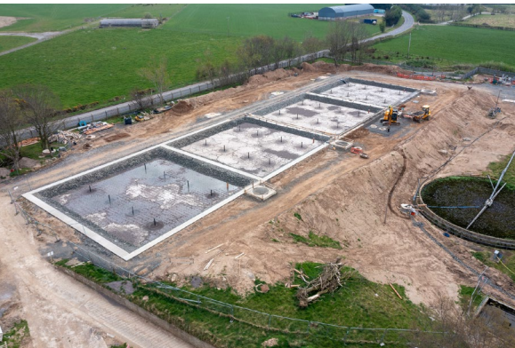
Construction of reed beds at Aghanloo wastewater treatment works, County Derry/Londonderry.
