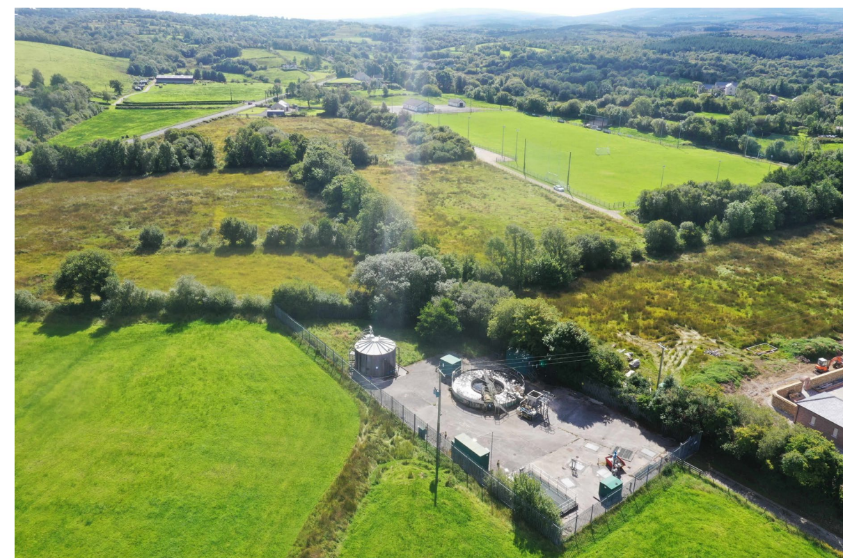
Garrison wastewater treatment works, County Fermanagh which is due to be replaced with a sustainable solution under the PEACEPLUS programme.
