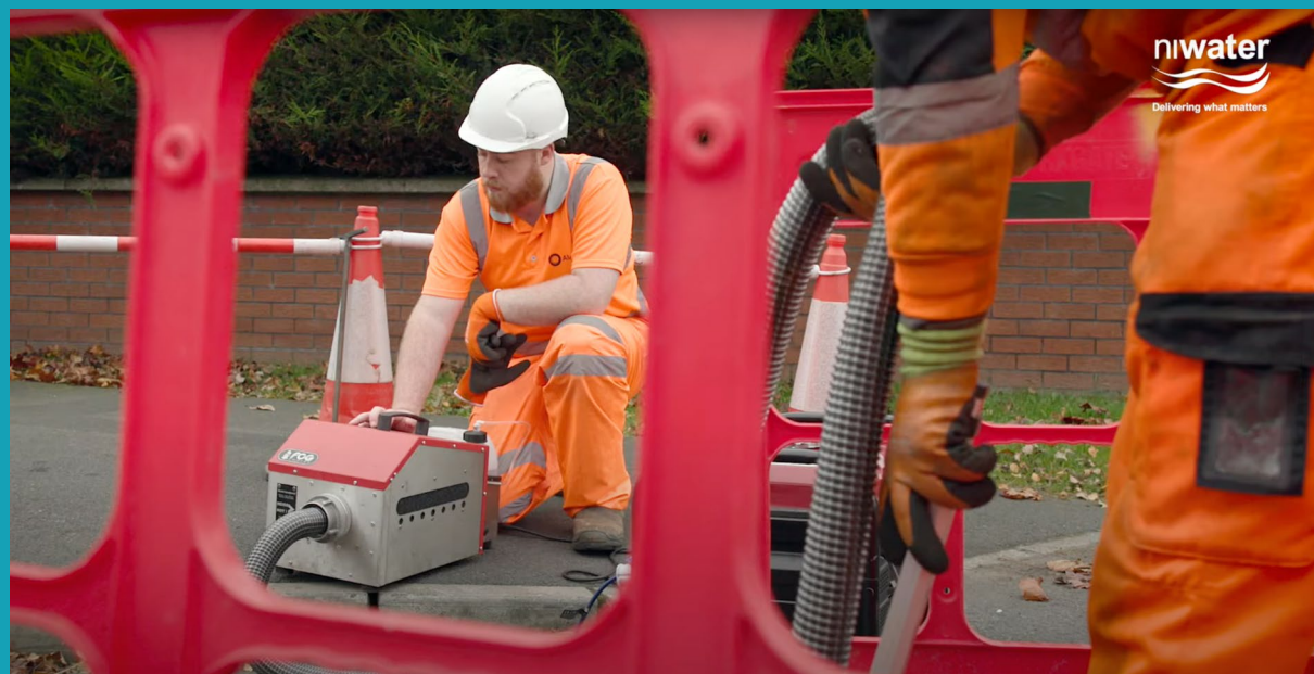
NI Water staff member using FOG technology to identify sewer misconnections.
