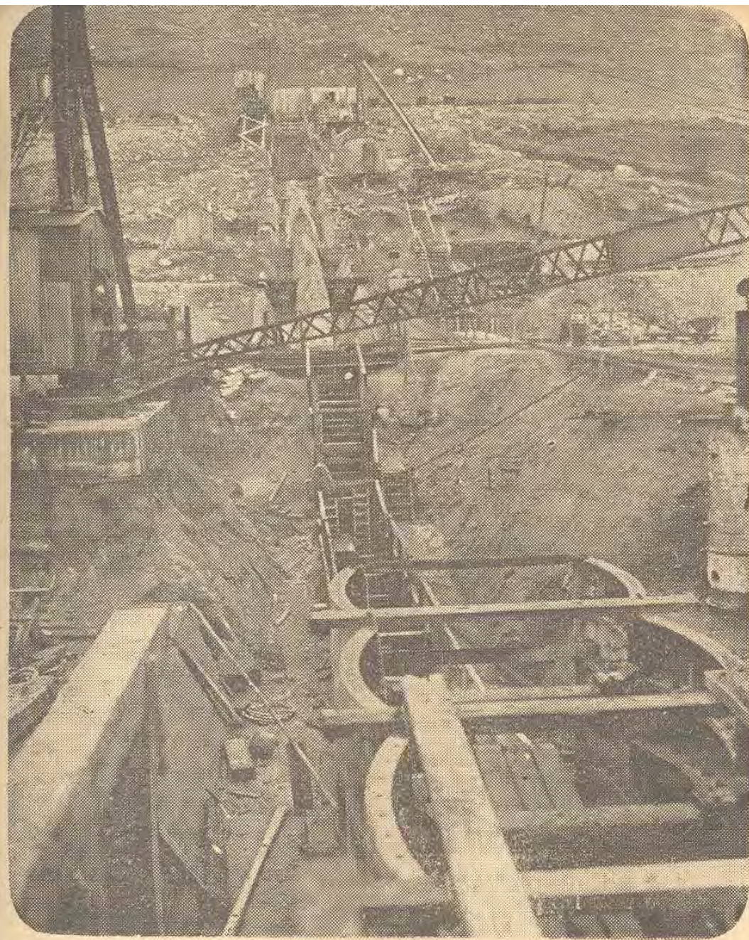
A GENERAL VIEW OF THE TRENCH EXCAVATION SHOWING THE CAST IRON LINING SEGMENTS.
