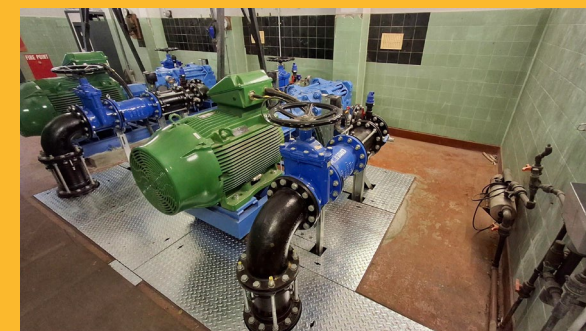
Pump replacement work at Whiteabbey water pumping station, County Antrim.
