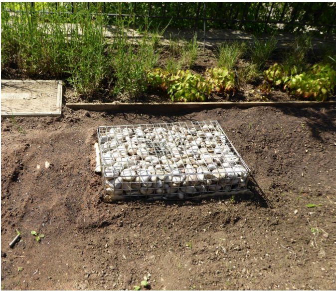
Image: Completed flow control in stone-filled filter basket before planting
