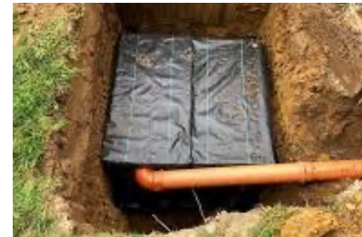
Image: Soakaway being installed
