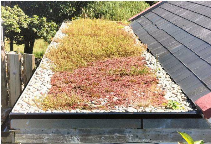
Image: Green roof installed on an extension
