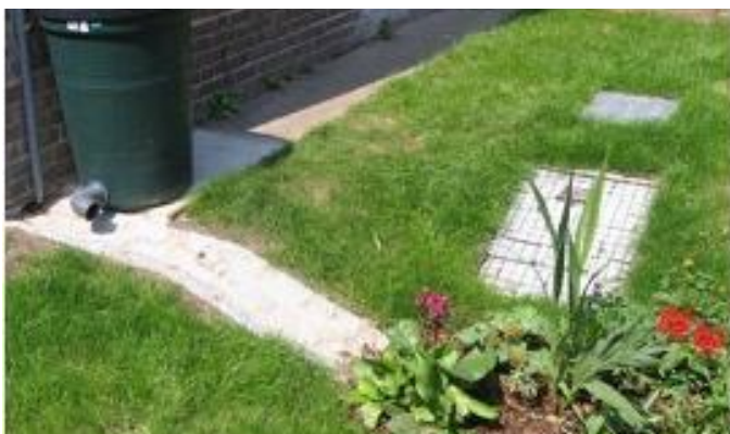
Image: Downpipe directed through water butt and then onwards to the rain garden.
