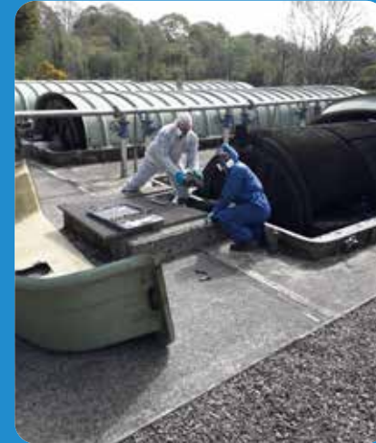
Mechanical and electrical operatives carrying out repairs
