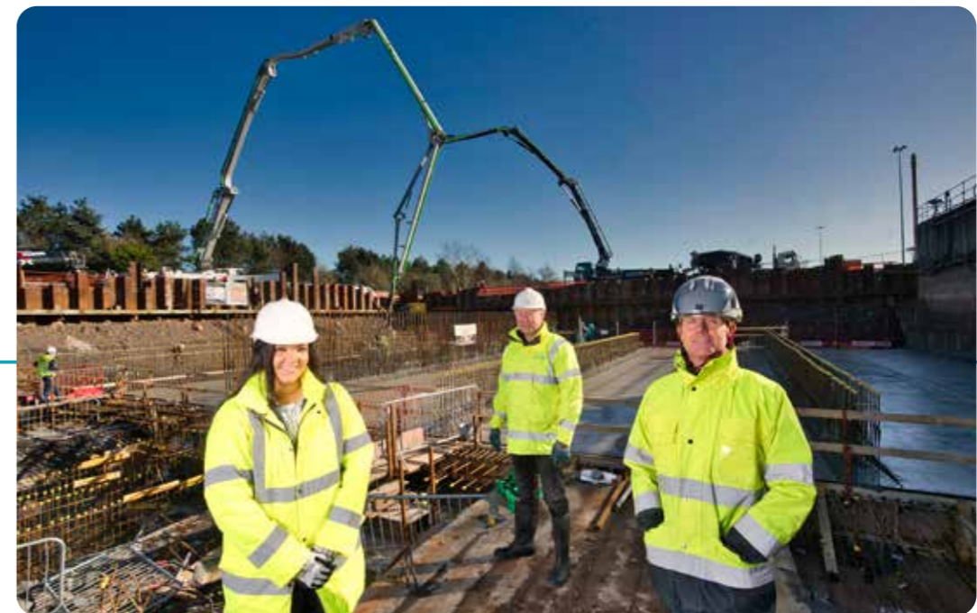
Construction of new treatment tanks at Belfast wastewater treatment works
