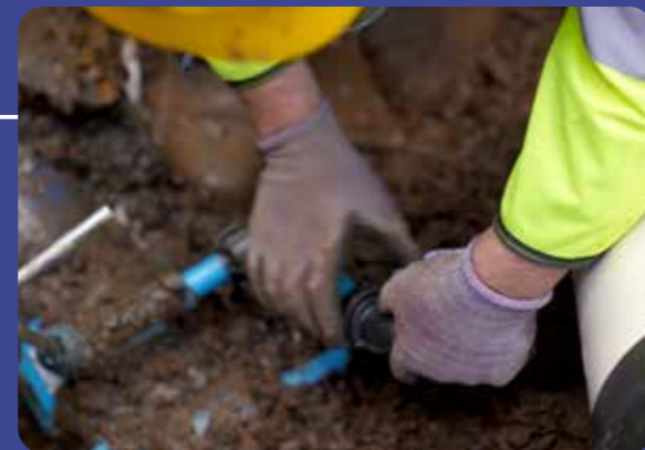
Repair to a burst pipe
