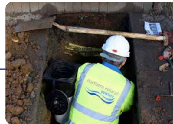
NI Water staff repairing supply interruptions
