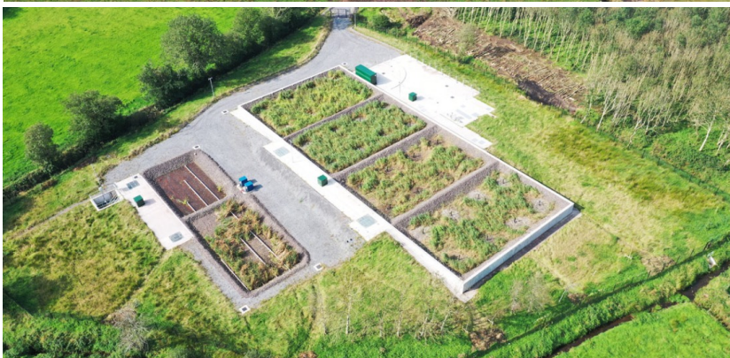
Clabby WwTW: September 2020 - Courtesy of BSG Civil Engineering Ltd
