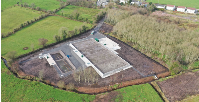
Clabby WwTW: February 2019 - Courtesy of BSG Civil Engineering Ltd
