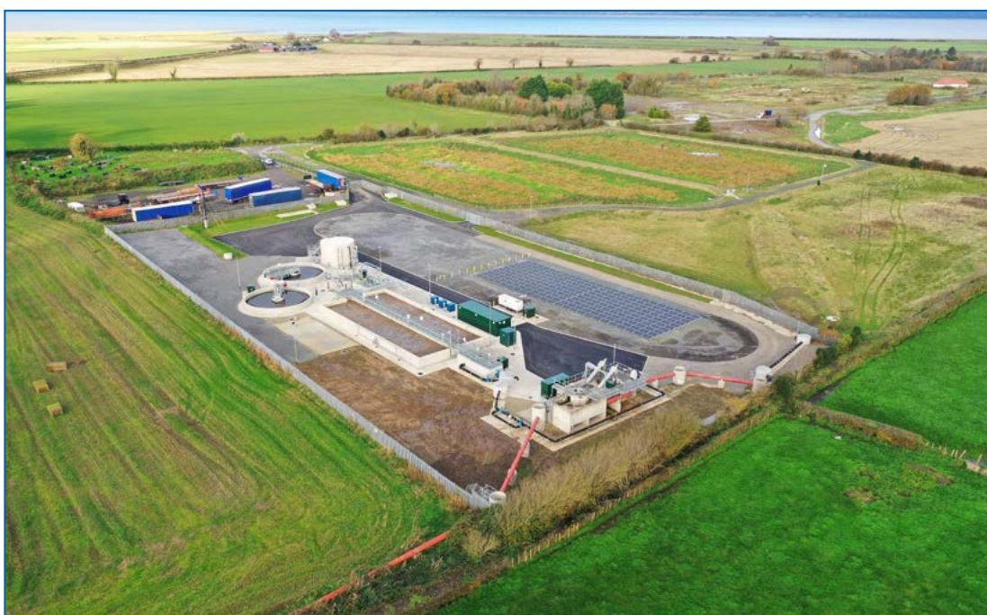
Ballykelly wastewater treatment works, County Derry/Londonderry.
