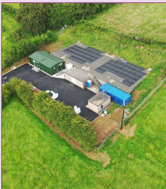
Moneymore Borehole in County Derry/Londonderry.
