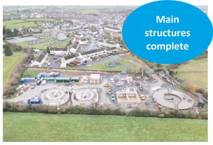
The main concrete structures - including the two new circular Cyclic Activated Sludge System (CASS) tanks - are now fully constructed. Over **2000m**<sup>3</sup> of concrete and **200 tonnes** of rebar were used in the construction of the new structures on site.
