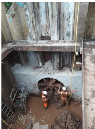
TBM Breakthrough
