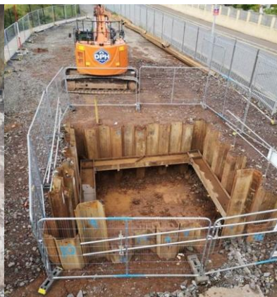
Preparation of Tunnelling Pit
