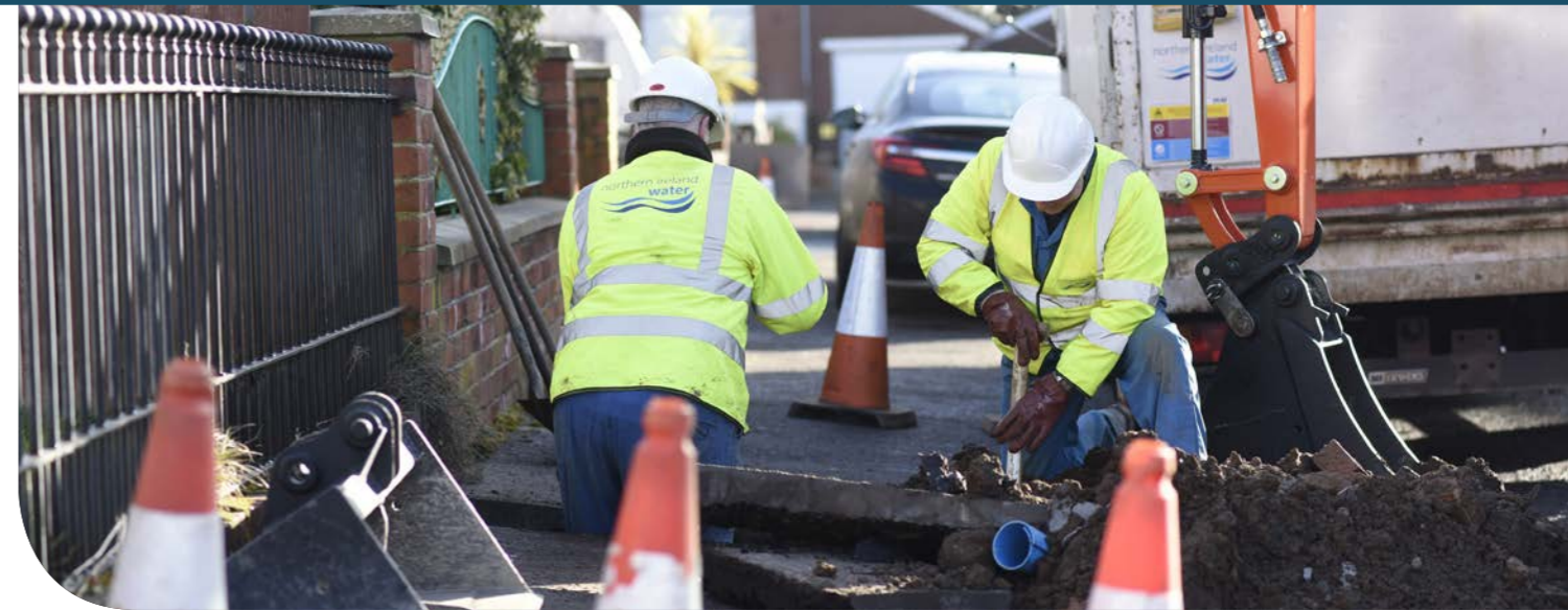
NI Water staff repairing a supply interruption.
