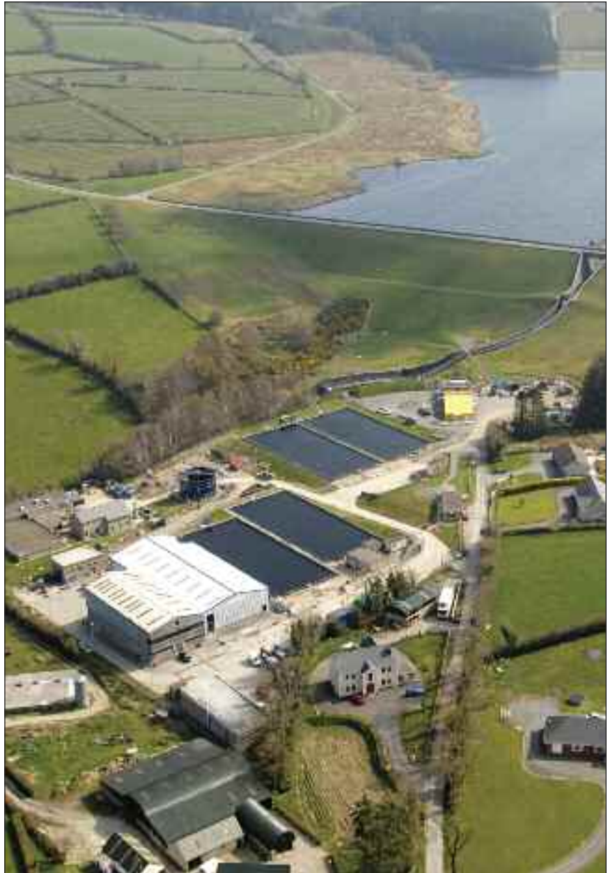
Seagahan Water Treatment Works
