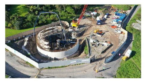
Construction of the tank is being carried out in cycles with periods of excavation works followed by concrete pours until the full 10m deep tank has been constructed. The next phase of rock breaking/excavation work is due to get underway in November.
