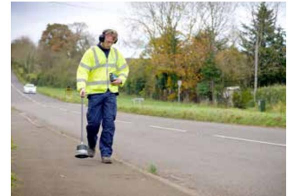
Detecting leaks using a ground microphone.
