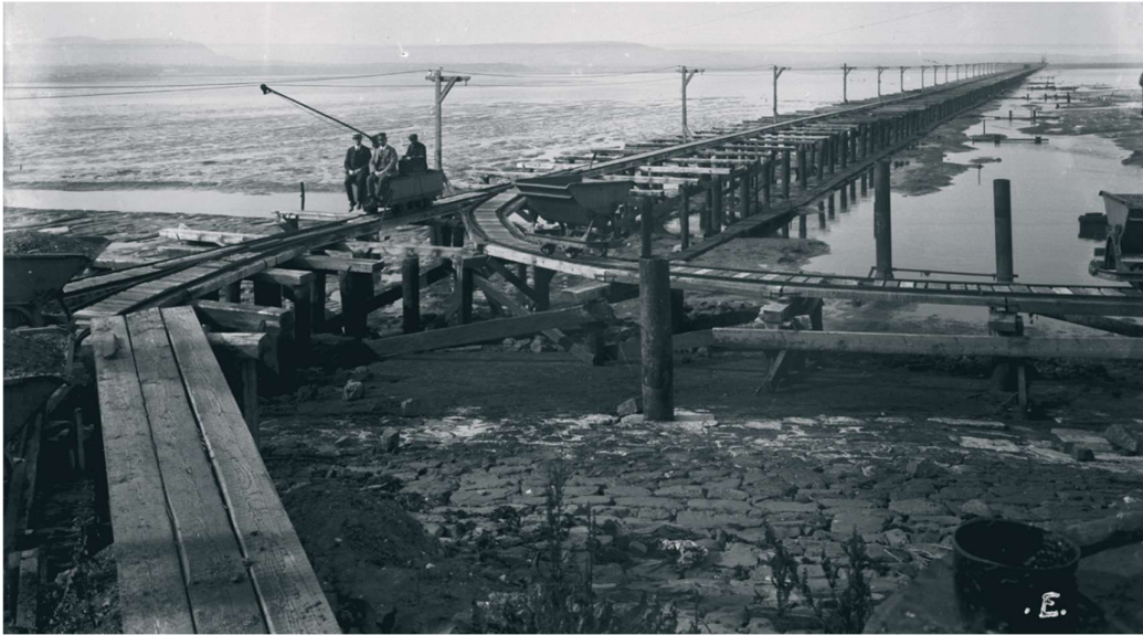
Figure 11: Belfast WwTW Sea Outfall During Construction (1913 to 1933) Photo sourced by NI Water from National Museums Northern Ireland (NMNI)
