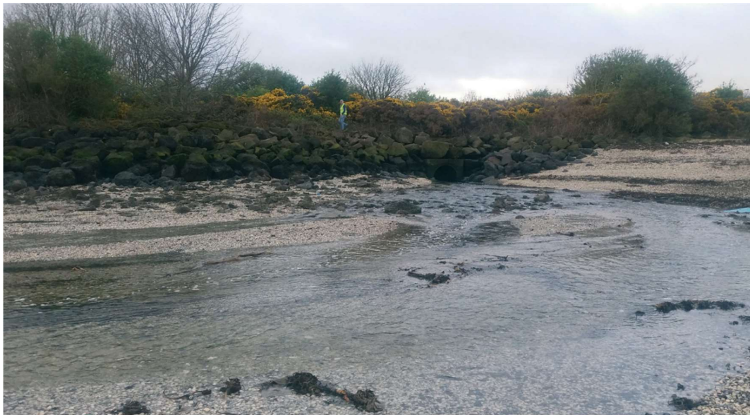
Figure 15: Whitehouse WwTW Discharge Headwall (temporary in 1977)
