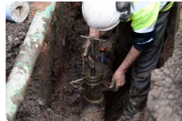
Lead communication pipes being replaced
