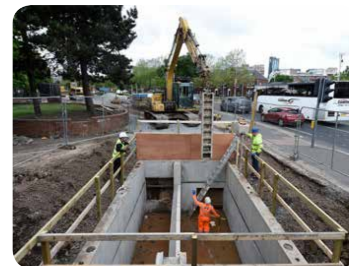
Storm water separation in Belfast city centre
