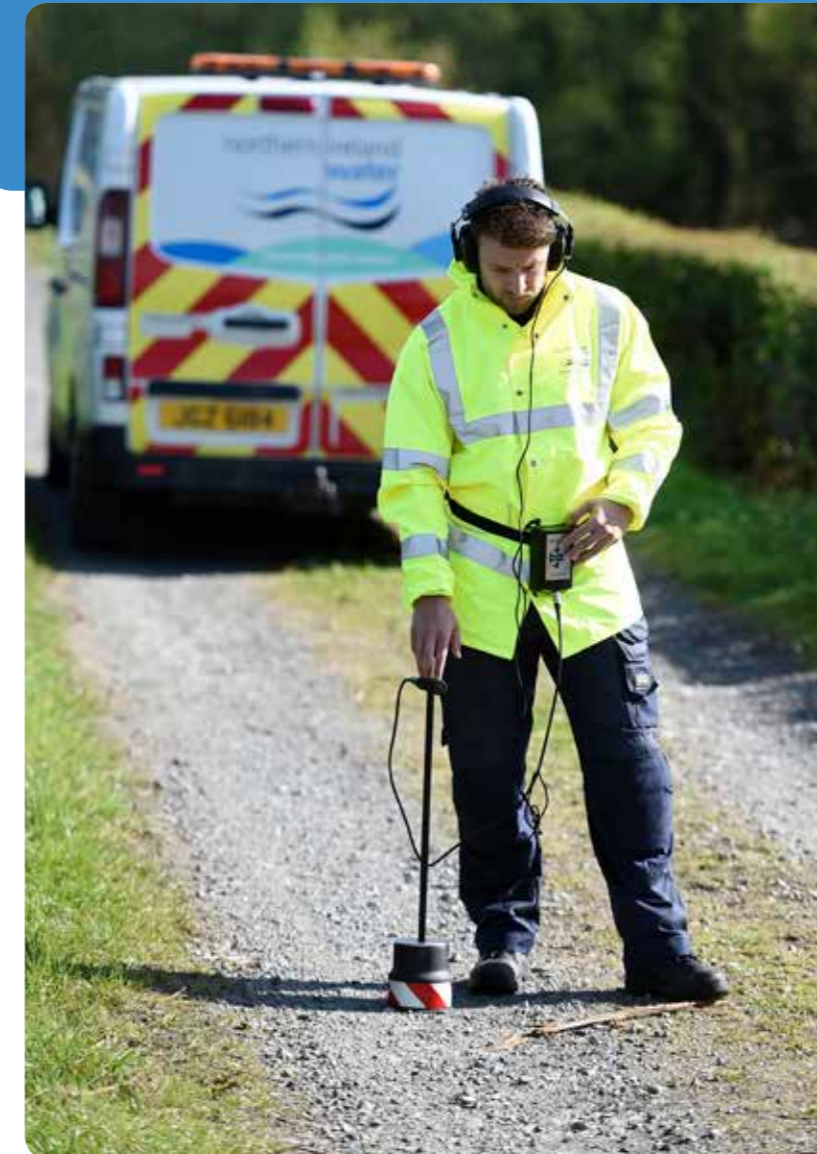
Leakage detection in Omagh, County Tyrone
