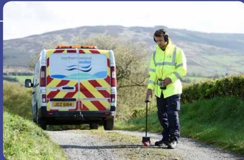
Leakage detection in Omagh, County Tyrone
