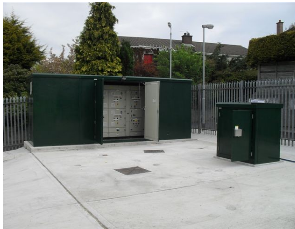
Photograph showing upgrade of a larger pumping station site
