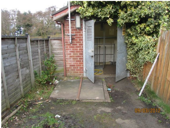
Typical wastewater pumping station due for refurbishment
