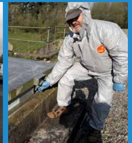
Service reservoir inspections carried out by the water production team
