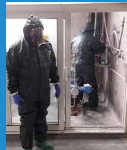
Water treatment operatives working on pumps
