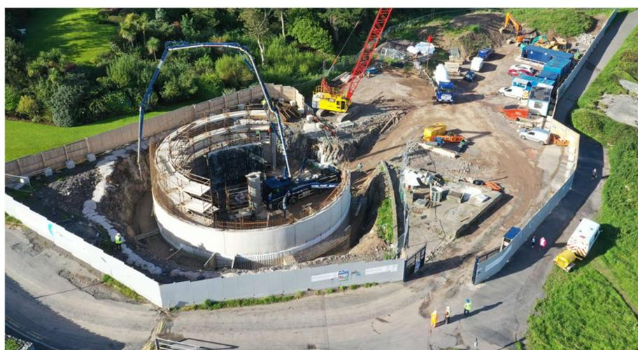
Construction of the tank is being carried out in cycles with periods of excavation works followed by concrete pours until the full 10m deep tank has been constructed. The next phase of rock breaking/excavation work is due to get underway in November.
