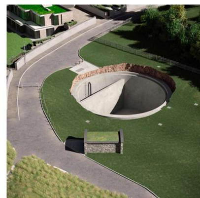
Once the tank is fully buried the area will be landscaped. There will be a concrete surround placed around the manholes to protect the covers and provide a hardstanding for maintenance operations. The only above-ground structure at the Brompton Road site will be the control building for the pumping station, which has been designed to resemble an old boat house with natural stone cladding to blend in with the natural environment.
