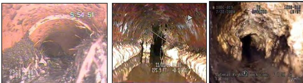
For regulatory reporting, silt, fat, roots debris are all classed as a blockage. However, it is important that the actual cause of the blockage is recorded within the incident record. The response to each of these might require a different solution. For example, a persistent fat problem may require trade effluent control or persistent siltation problems may need to be added to the de-siltation programme for that area.
