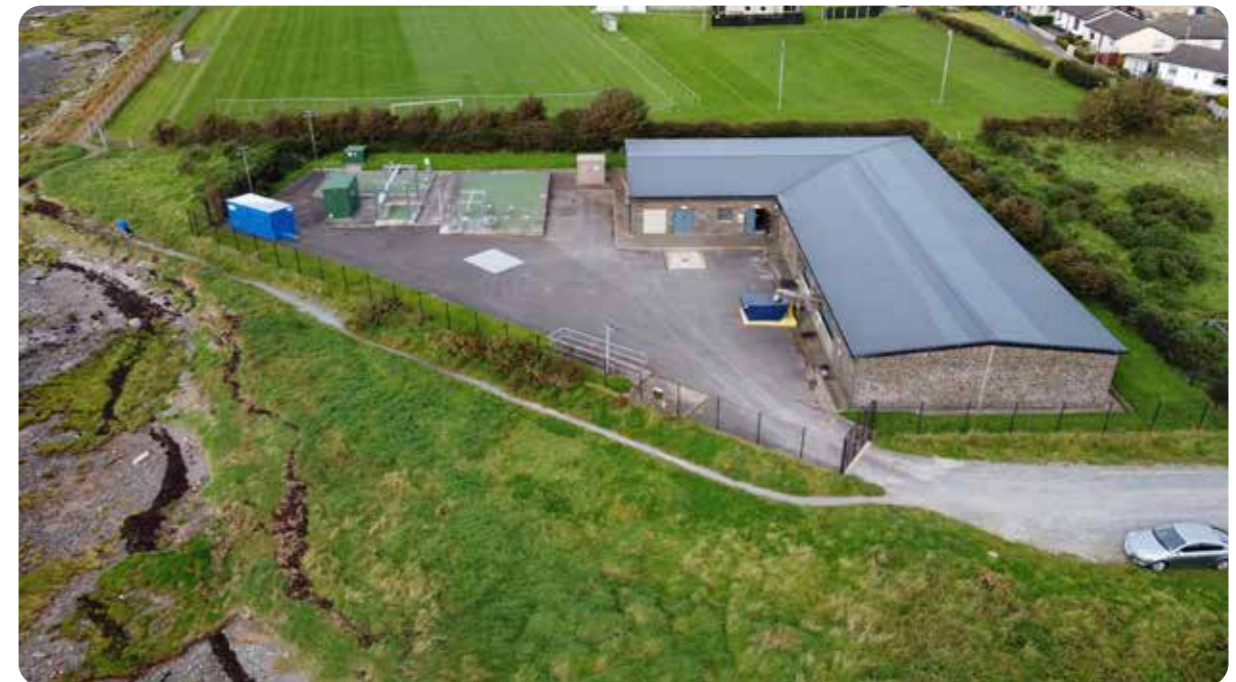
Greyabbey wastewater treatment works, County Down
