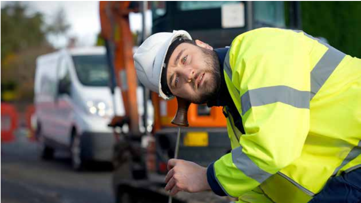
Networks Leakage Technician, using a listening stick to detect a leak.
