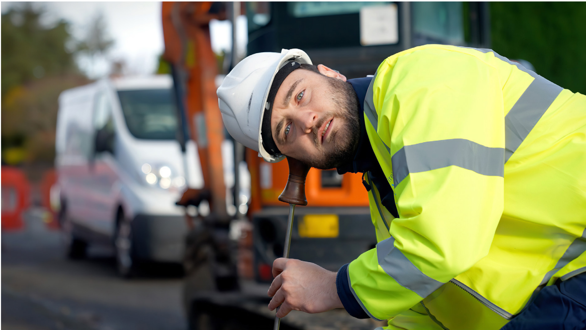
Networks Leakage Technician, using a listening stick to detect a leak.
