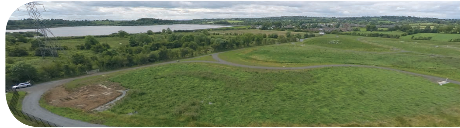
Natural wetland treating used water at Stoneyford, County Antrim. We received a prestigious international 'Green Apple' environmental award in recognition of our work to construct a natural wetland for treatment of used water in Stoneyford, near Lisburn, County Antrim. The Stoneyford site is a flagship project for NI Water to produce an industry-leading example of how treatment can be integrated into and complement the local ecosystem. The approach requires less capital investment, uses less energy and chemicals, and requires less maintenance compared with traditional solutions. Following the success of Stoneyford, we opened a second wetland at Castle Archdale, County Fermanagh.
