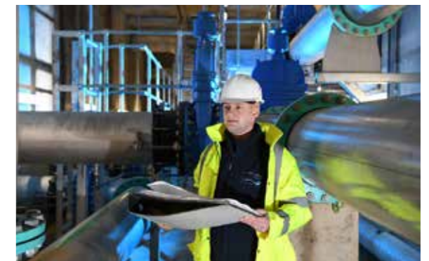
The new Lough Fea service reservoir, County Tyrone
